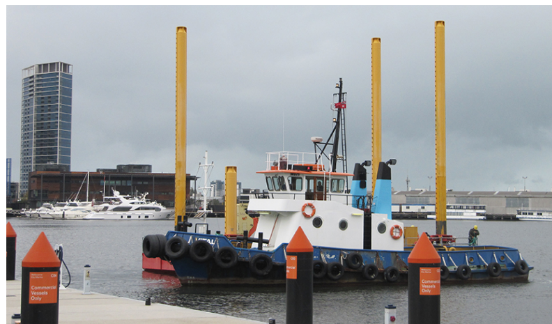
Vital positioning Korevaar's Jackup Barge 1 at Docklands, Melbourne
