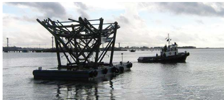
Barge 74 transporting roof trusses for Southern Cross Station from Geelong to Melbourne
