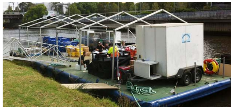
Temporary kitchen facility for use at a river-side wedding reception, under construction on Barge 73
