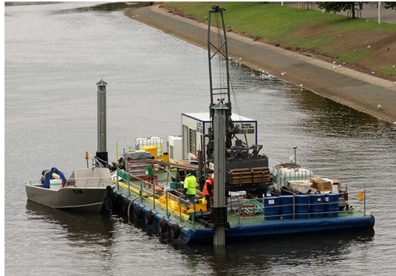
Barge 73 fitted with spuds and carrying out geophysical testing in the Yarra River, Melbourne
