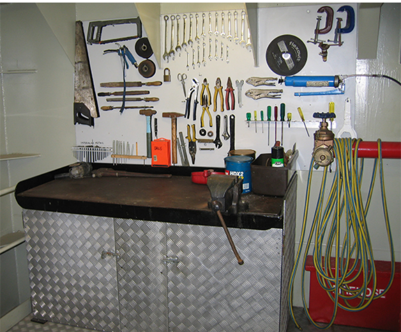
Workbench in forward pump room
