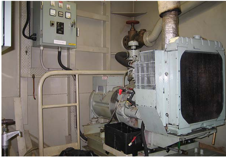
Aft pump room including 27 kVA 3 phase genset
