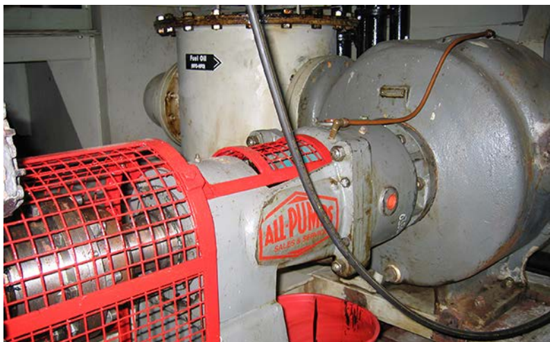
HFO cargo pump in aft pump room
