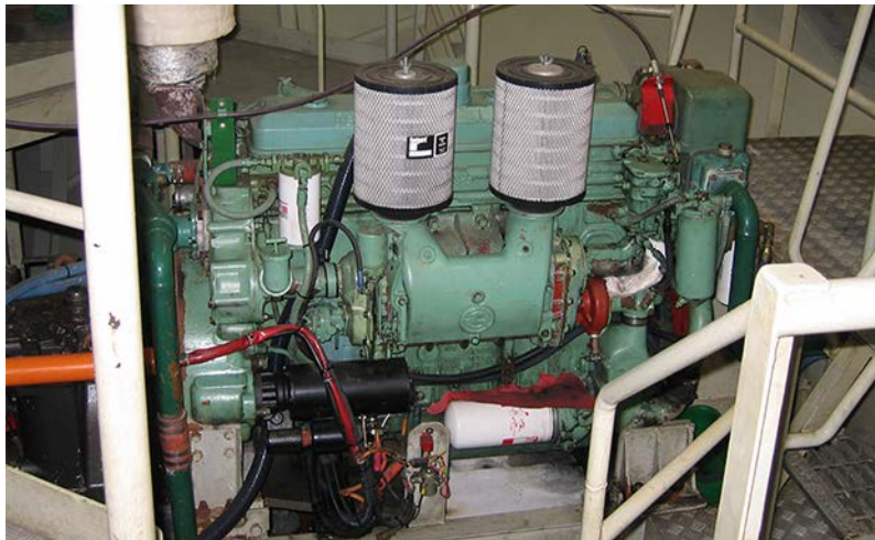
HFO cargo pump engine in aft pump room
