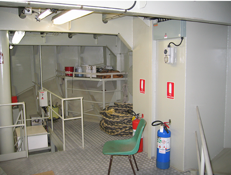
Forward pump room
