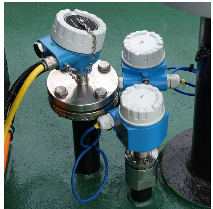
Temperature measurement fitted to each of the 6 cargo tanks
